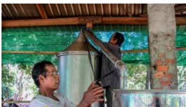
Step 2.2: tanks' connection
