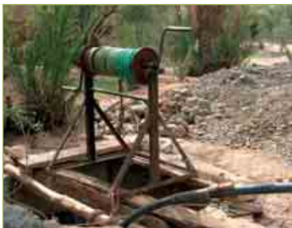
Building a well, Morocco
