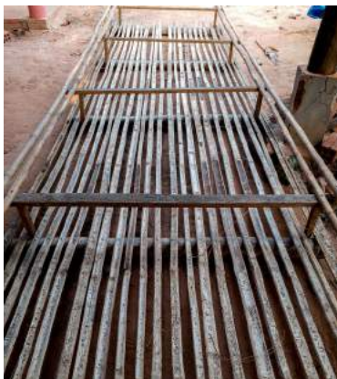
Step 2: Bamboo structure
