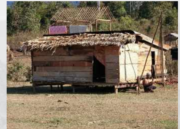
Wooden walls and straw roof house in Navang village
