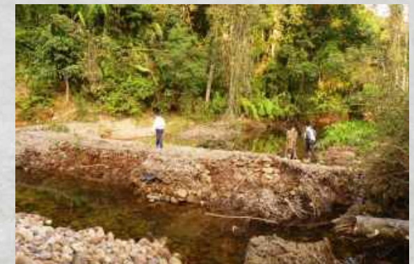
Gabion basket dam in Nameoy
