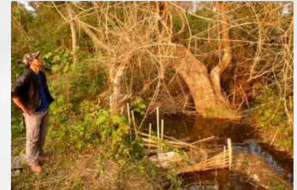
Individual earth weir in Navang
