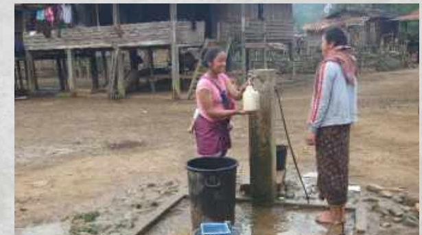
Water supply system on Korbong hamlet
