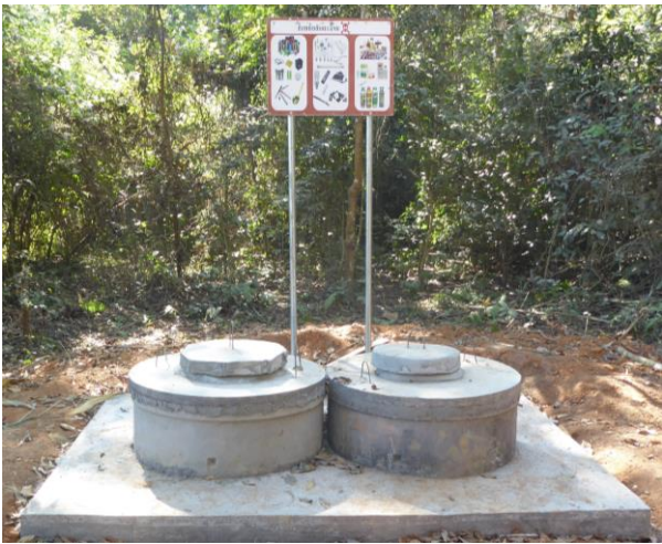
Hazardous waste pits in Samsoum village
